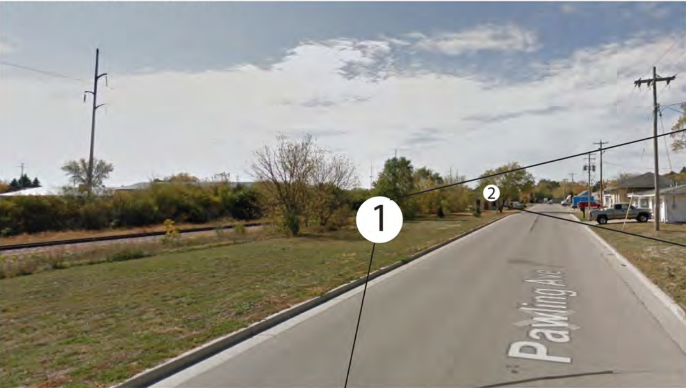
STREET VIEW (LOOKING WEST)
